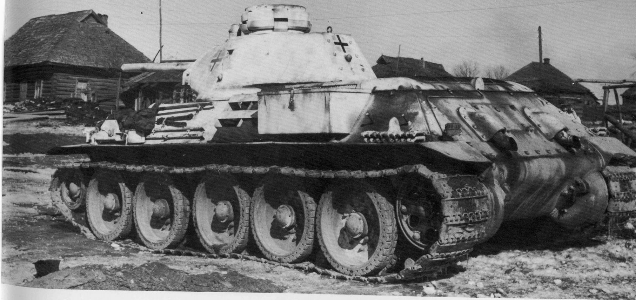
A T-34 (1941 model) with a German commander's cupola added, in use by the 98th Infantry Division. The tank is also equipped with German camouflage light, auto jack and tools. (BA)
