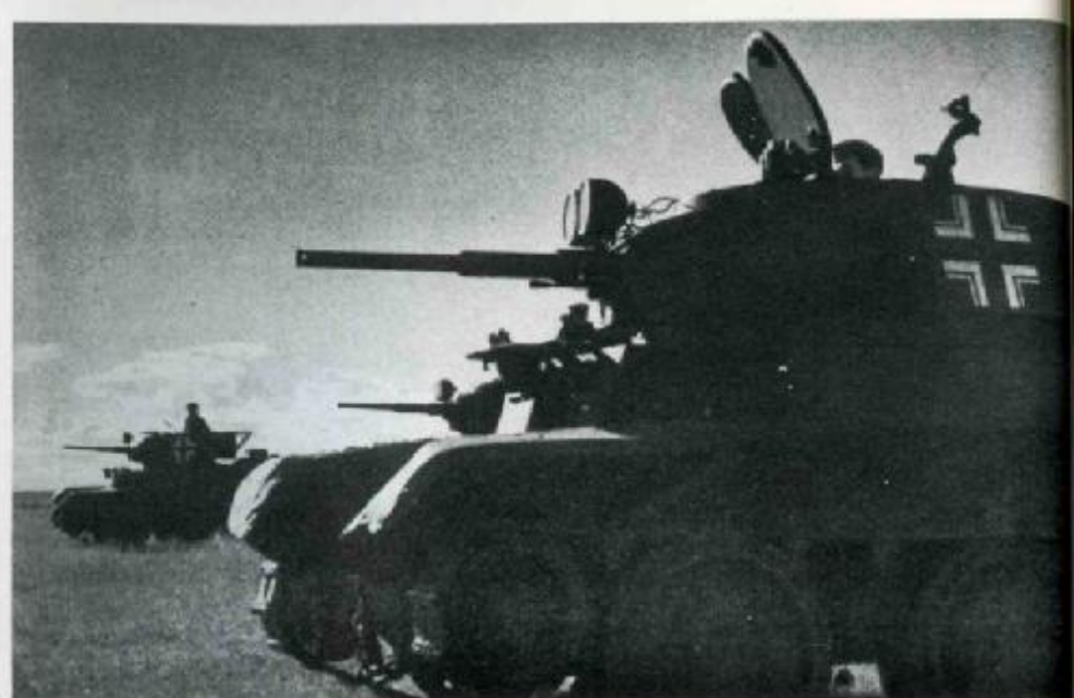
Three BT-7 tanks with very noticeable German crosses painted on. These were three different versions of the Type BT-7. In front in the picture, the last production type BT-7 M (also called BT-8) can be seen, with one oval and one round turret hatch as well as mountings for an anti-aircraft machine gun (1939 type). In the middle is the BT-7 (built in 1937), and at the rear a Type BT-7TU (built in 1935). The suffixed TU indicates that it is a command tank, thus it is equipped with a frame antenna. All three tanks have their original Russian shooting spotlights mounted. (Frank)
